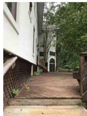
side deck/next to swim. pool
