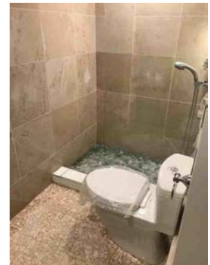
full bath# 1 (basement level)
