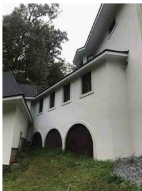
connecting way to garage
